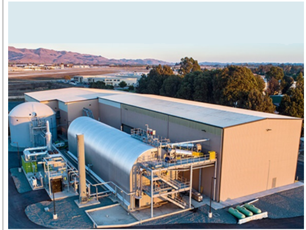
Anaerobic Digestion Facility in San Luis Obispo, California
