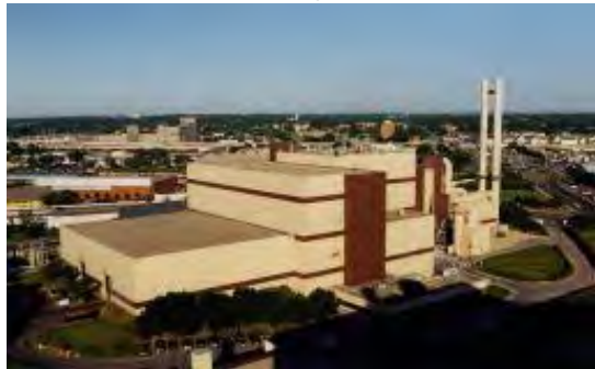
Hennepin Energy Recovery Center
