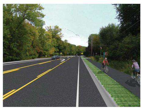
**3** Near Russell Ave – Overhead Utility Crossing Burial Road realignment, trail, turf boulevard, curb/gutter, reduced aboveground utilities
