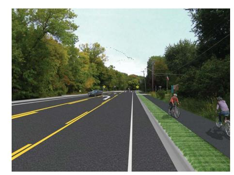
**2** Near Russell Ave – Additional Trails and Sidewalks Road realignment, trail, turf boulevard and curb/gutter
