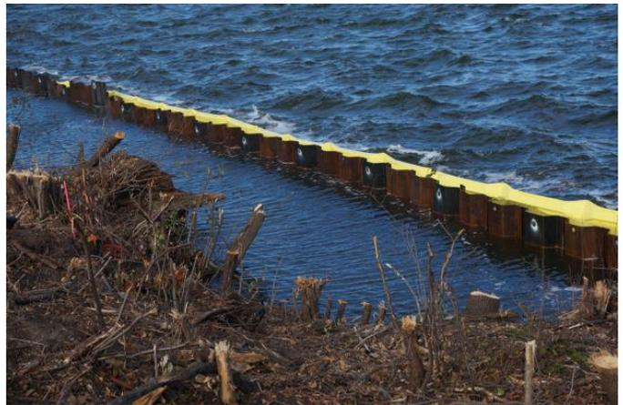
*The steel walls are necessary to provide a perimeter so that water can be removed from within the work area.*
