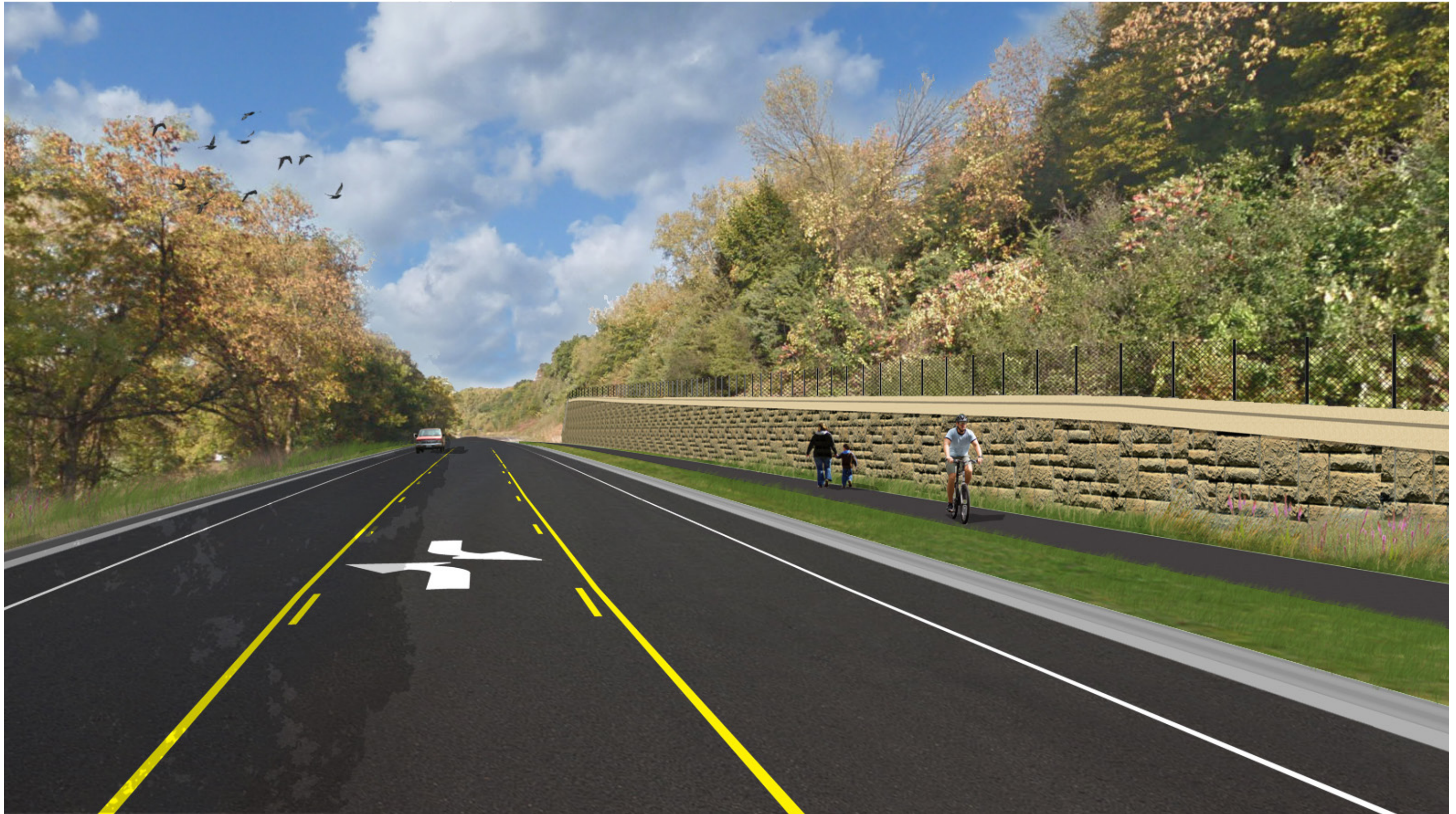
Driver's Perspective - Looking West at Station 122+00, Adjacent to Wall 7 (Cast-in-Place Concrete)
