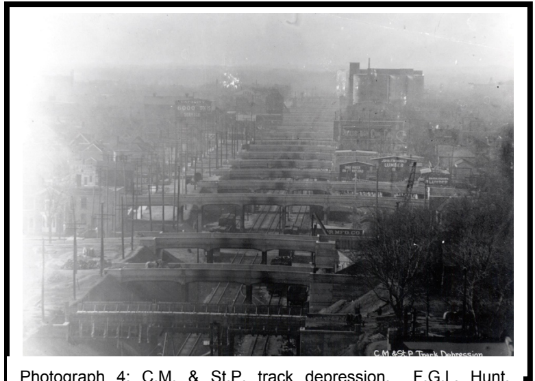
Photograph 4: C.M. & St.P. track depression. F.G.L. Hunt, Engineer. From Minnesota Historical Society Album #212, The C.M. & St. P. Track Depression Construction Project, ca. 1900. Negative #87062.
