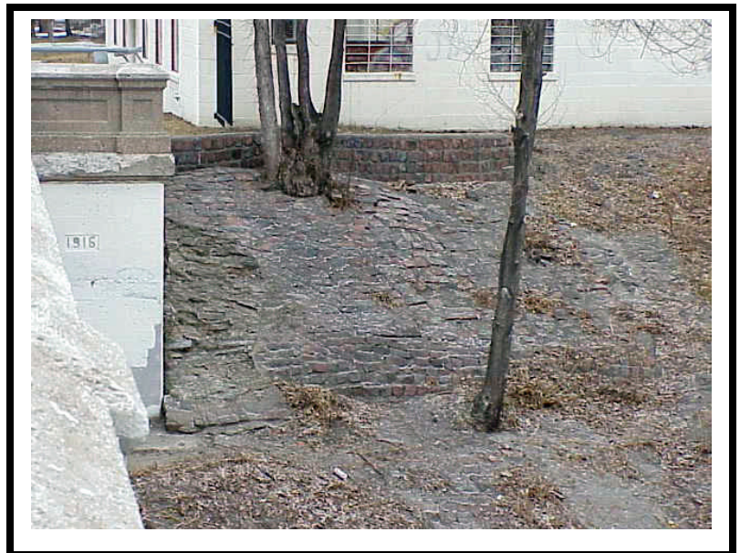
Photograph 8: Typical granite block retainer.
