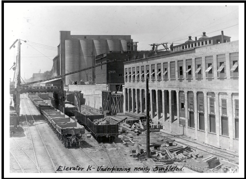
Photograph 3: Sheffield Elevator "K"- underpinnings nearly completed. Photo from Minnesota Historical Society Album #212, The C.M. & St P. Track Depression Construction Project, ca 1900. Negative #87069.
