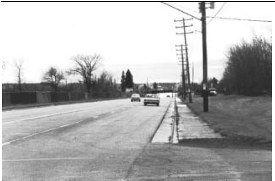
Example of a basic roadway with no special accommodations for bicycles
