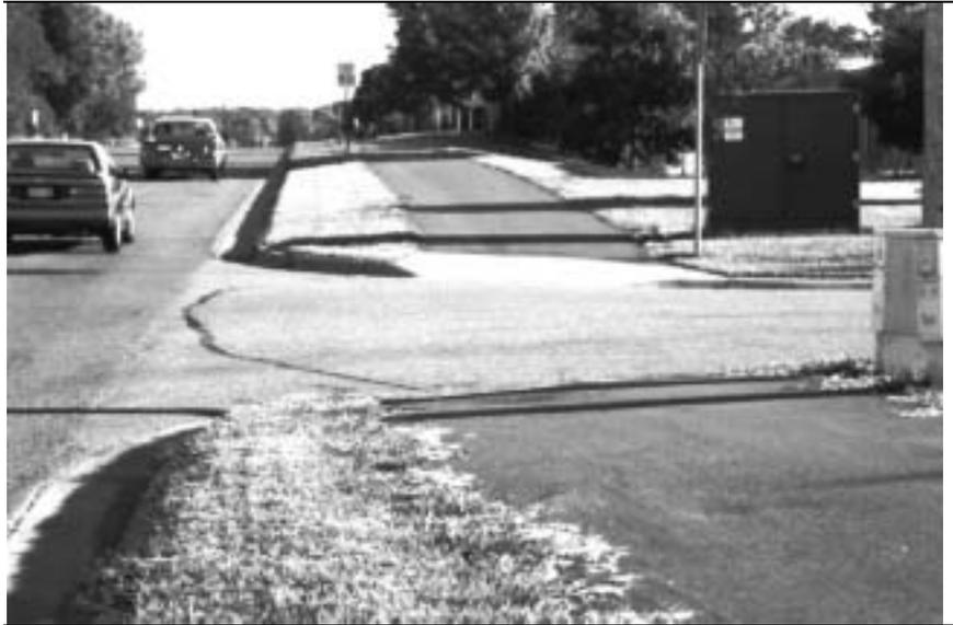
**Basic Roadway** accommodations means that due to design and / or right-of-way constraints, bicycles must share road space with motorized traffic. Under this situation, the county routinely removes obstacles and hazards to bicycle travel along the roadway edge. In some cases where adjacent sidewalks and occasional bicycle usage exists, a widened lane may be provided to provide refuge space and vehicle reaction distance.
