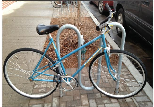
**Discouraged — Undulating or snake:** Provides only one point of contact and does not accommodate the intended number of bikes. It often is used incorrectly.
