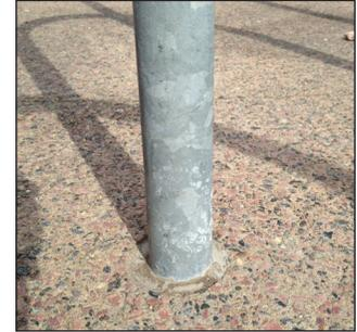
**Recommended:** Bolt each leg or base securely using wedge anchor bolts or tamper-proof spikes (left); or embed legs or base in concrete or bituminous.
