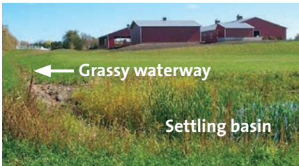
A clean water diversion carries clean water around potential contaminants like bare soil and manure.
