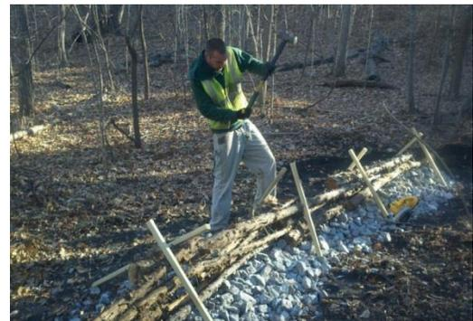
*The county and the Minnesota Tree Trust installed check dams on a conservation easement in Minnetrista to control stormwater runoff directed towards a rare bog downstream.*
