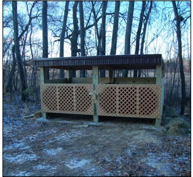
Example of a compost bin for non-production or small site livestock facility.
