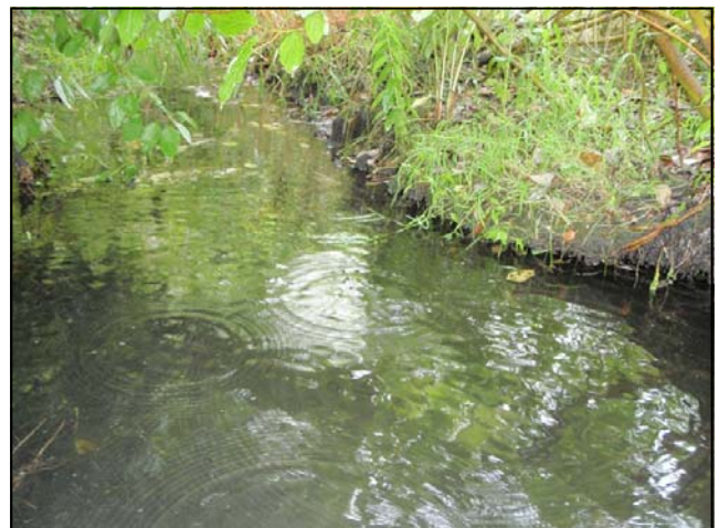
Channel Scour at outlet to Pond 1a.
