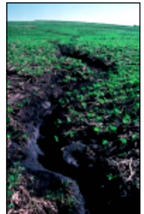
Example of gully erosion that is commonly observed in this watershed.
