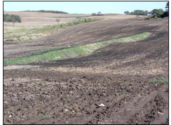
Example of a typical water and sediment control basin layout.
