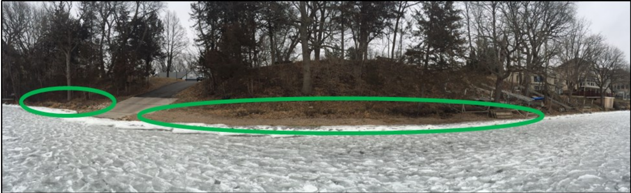
Figure 15U: The erosion exists on both sides of the boat launch. It extends approximately 120 ft. to the right of the launch and 40 ft. to the left.
