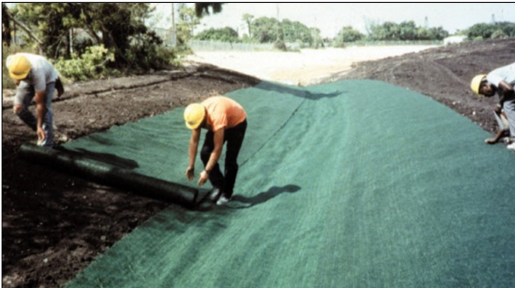
Figure 10U: Stabilization using manufactured synthetic products; Source: Contech Engineered Solutions
