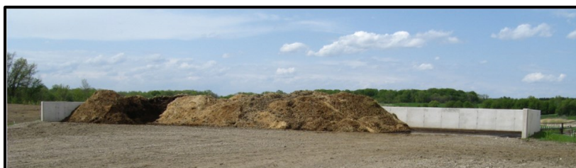
Figure 12R: Photo of aboveground concrete storage system for horse waste
