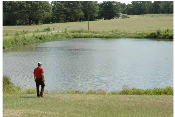
Figure 16R: Photo of constructed stormwater pond
