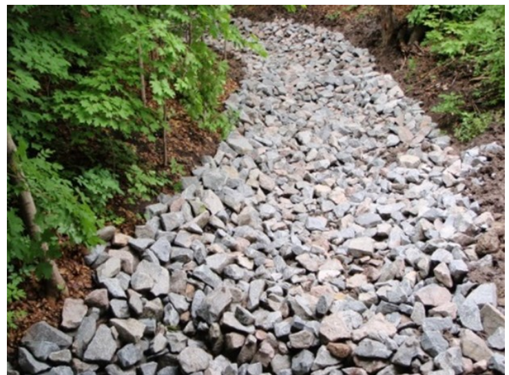
Figure 8R: Photo of rip-rap lined gully stabilization BMP
