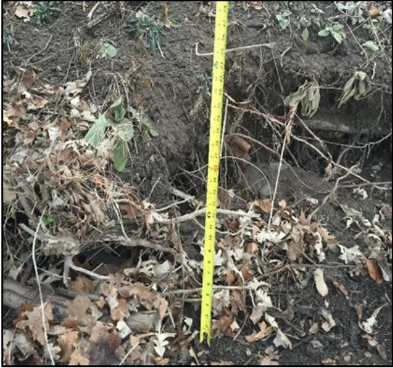
Figure 14U: Close up of the shoreline erosion
