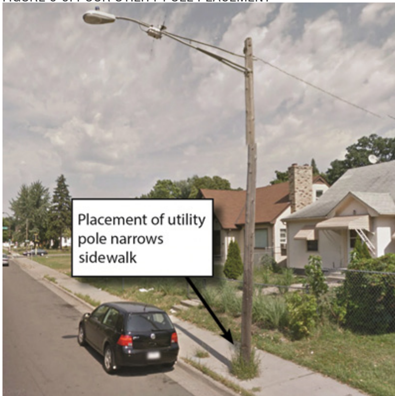
FIGURE 6-5: POOR UTILITY POLE PLACEMENT
