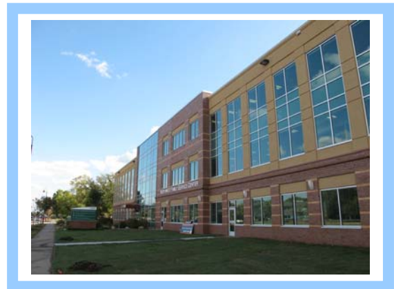
Northwest Family Service Center in Brooklyn Park
