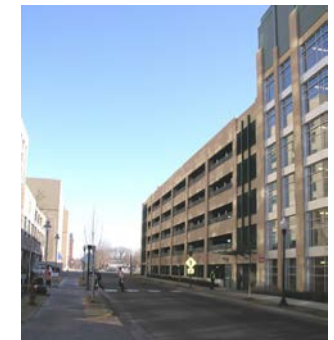
Parking Ramp on 10th Ave. Looking North
