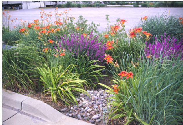
Small Rain Garden with Curb Cut
