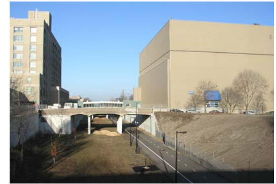
Greenway from 11th Avenue Looking West
