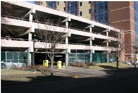
Parking Ramp on 10th Avenue
