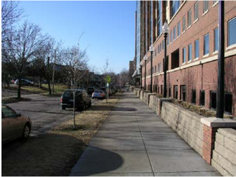
10th Avenue Sidewalk Along Abbott Northwestern Hospital Looking South
