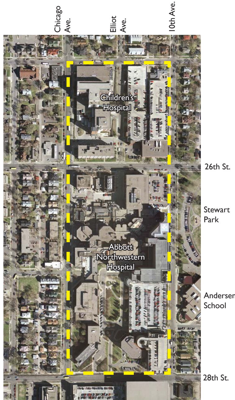
Aerial Photo of Hospitals Area
