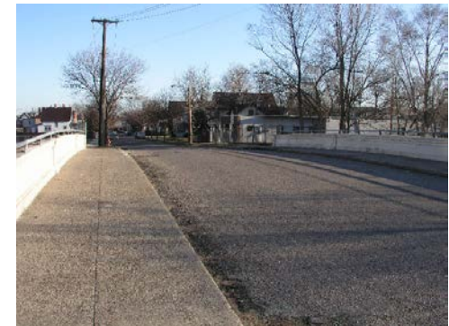
11th Avenue Bridge Over the Greenway Looking North
