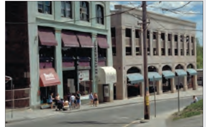
The parking ramp (building on the right) takes direct cues from surrounding architecture.
