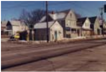
Deteriorated properties are seen as a threat to Lowry Avenue
